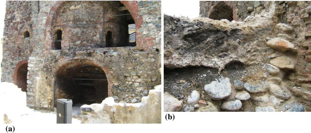
**Figure 1.** The remains of “Fornace Bianchi”(a) and the semi-coherent heap of lime (b)
